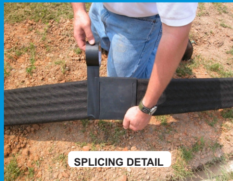
INSTALL AND TAPE FITTINGS
