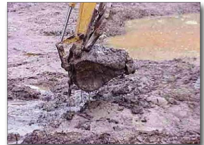
Figure 36. Removing stiffened sediment from a sediment basin
