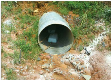
Figure 39. Polymer block in a construction site culvert
