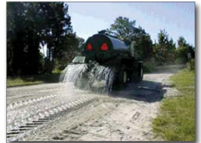
Figure 11. Water truck applying dissolved polymer flocculant
