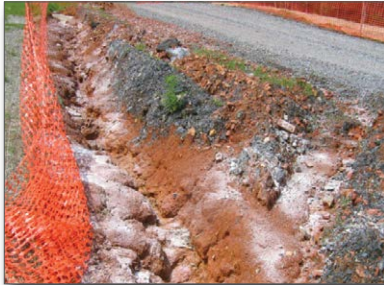
Figure 38. Eroding gully on a construction site
