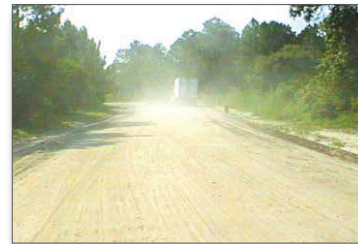
Figure 12. Road dust before applying polymer flocculant
