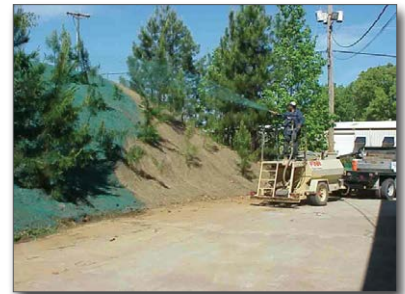
Figure 5. Hydroseeding the slope
