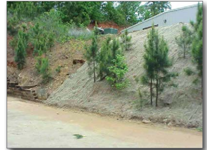
Figure 4. Slope covered with floc collection matting
