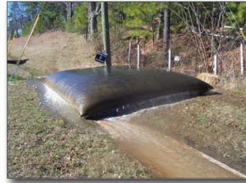
Figure 34. Sediment bag and its treatment ditch
