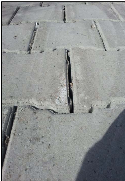
Steel Snow Plow Damage
