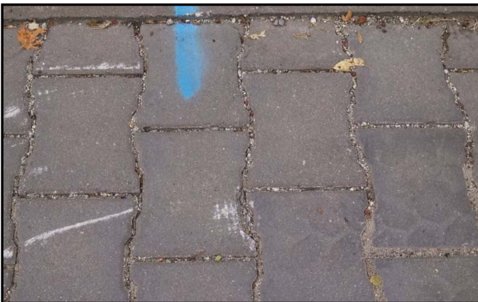
Photo 1 – PaveDrain needs to be maintained
