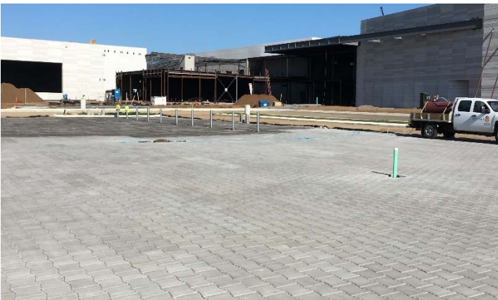
Sealant being applied on PaveDrain via Sprayer
