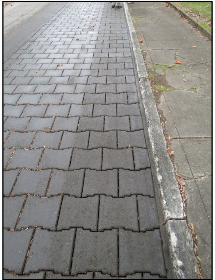
The 32" suction path is visible on the surface of the PaveDrain System after one pass of the Whirlwind.
