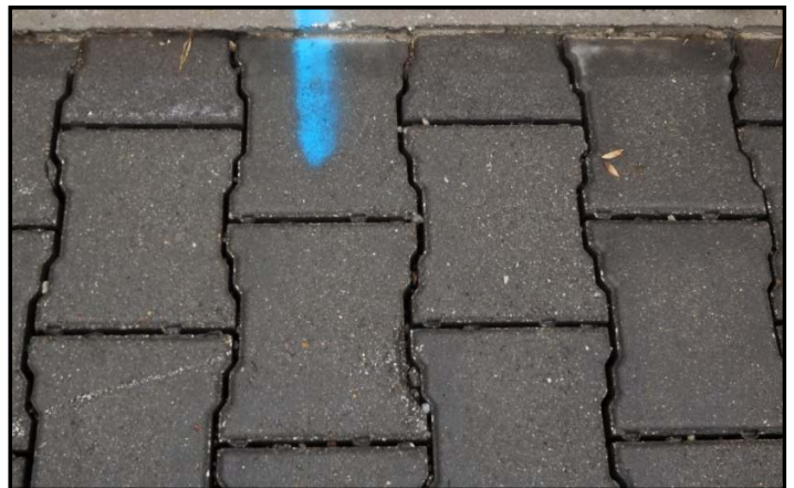
Photo 2 – PaveDrain following maintenance
