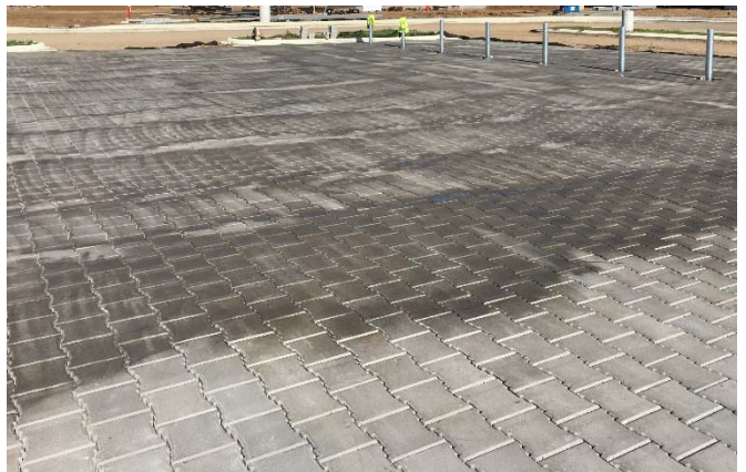
Close up immediately following sealant
