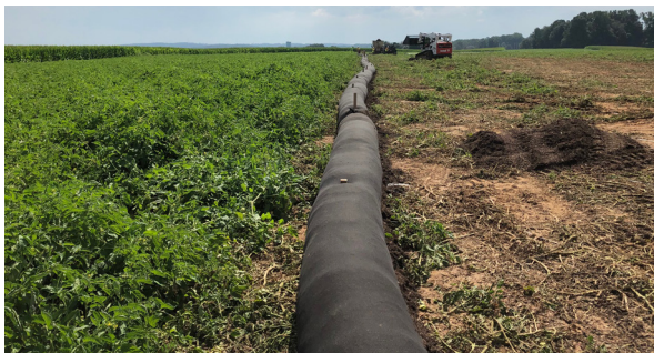
Filter sock used as perimeter protection on a pipeline project.
